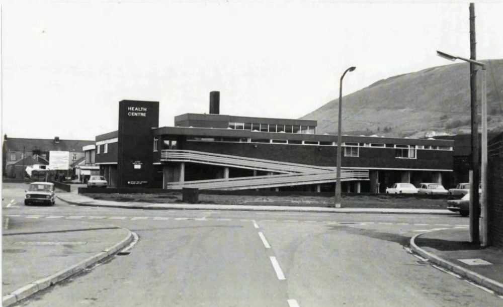
PLATE 12 Port Talbot - Aberavon Health Centre (14 G.P's)
