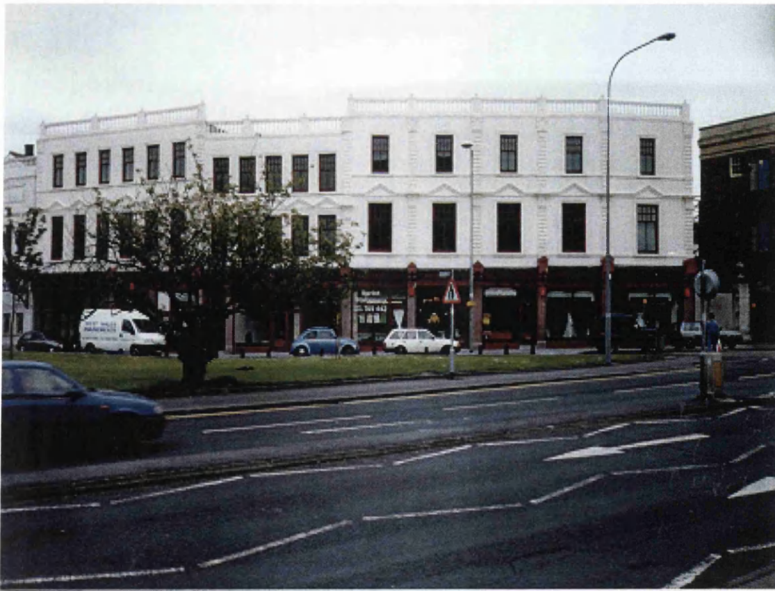
Plate 8: Lucania Buildings 1997 showing up-graded facade
