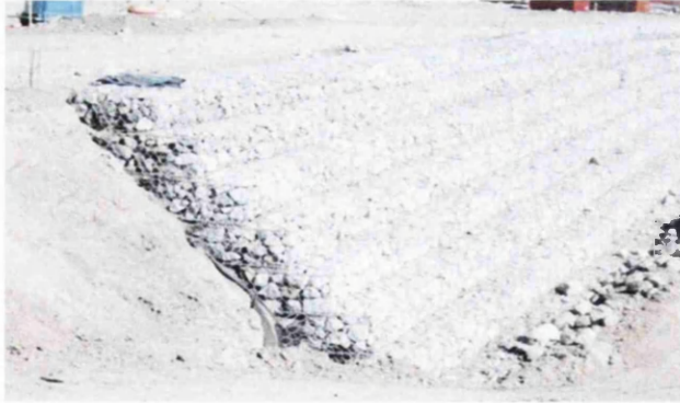
Figure 1.5. Downstream slope protection by gabion
