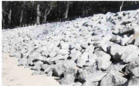
Figure 1.3. Riprap protection over a downstream slope
