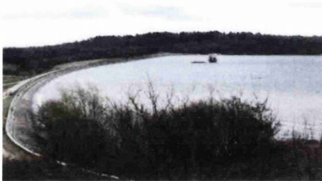
Figure 1.1. The dam at Bewl water in Kent, UK is an example of an embankment dam.
