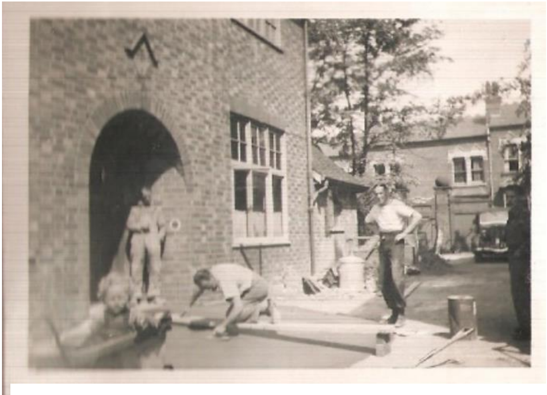
Laying the entrance ramp
