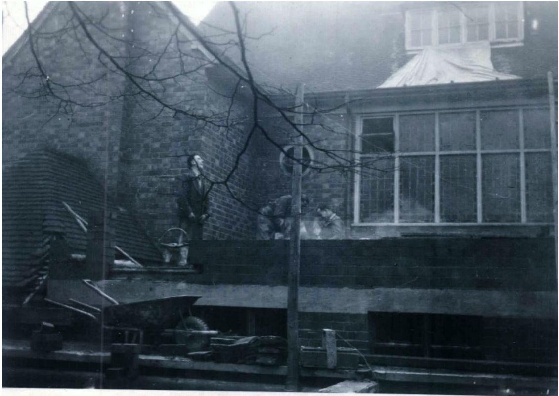
Roofing the cloakrooms
