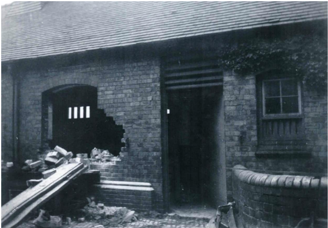
Adapting the stables to a treatment centre
