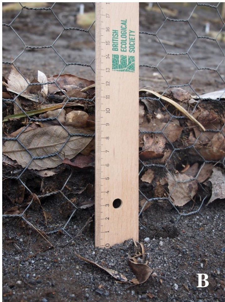
Figures 8.16A and B: Debris build-up along the fence at the bottom of the west-facing tailings slope at Nantymwyn, March 2019
