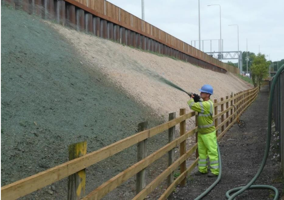
Figure 2.10: Hydroseeding a 45 ° railway embankment slope ( www.Salixrw.com )
