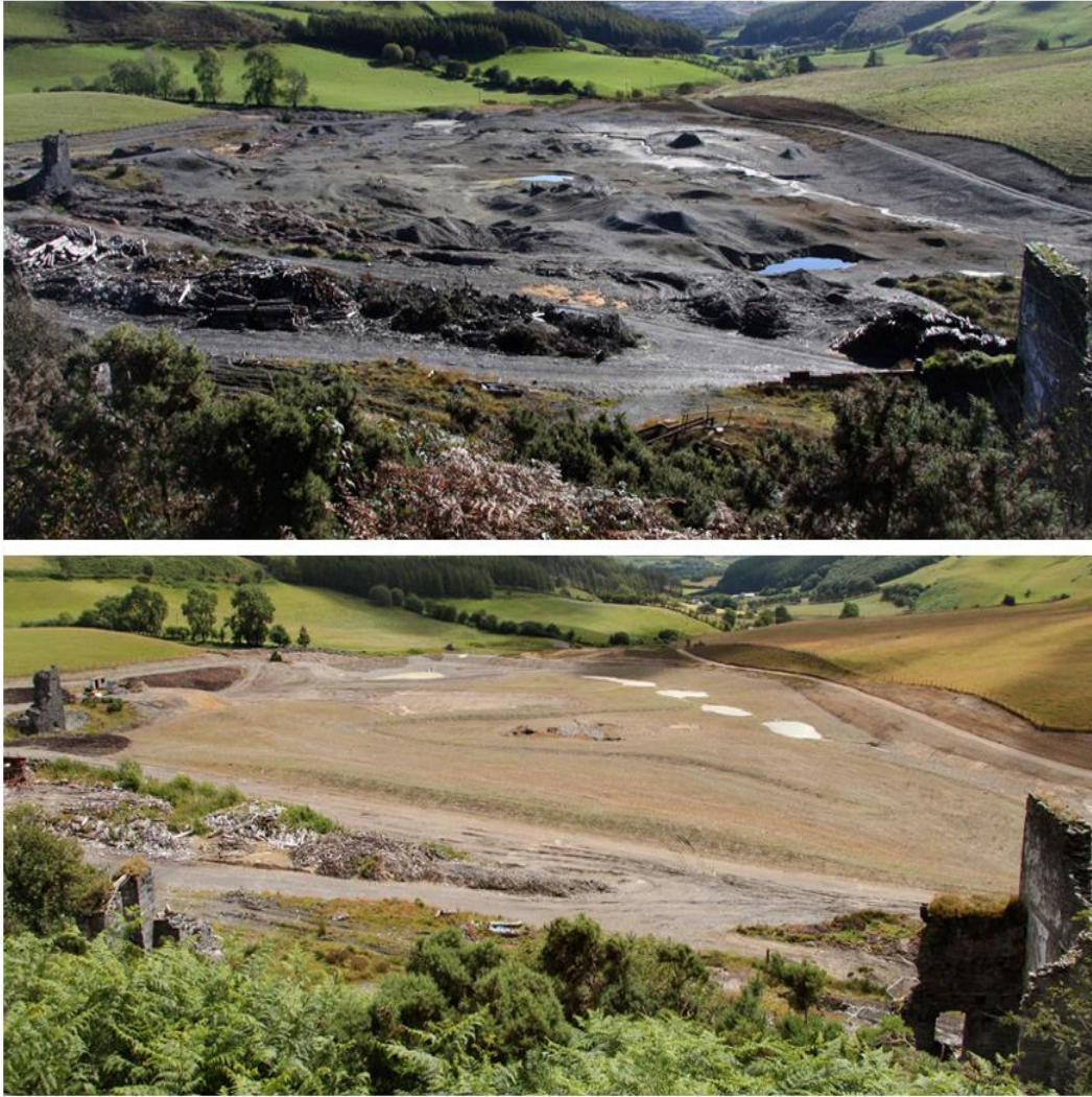
Figure 2.5: Frongoch Pb/Zn mine before (top, 2010) and after (bottom, 2016) a deep cap and cover system was applied (Edwards et al. , 2016)
