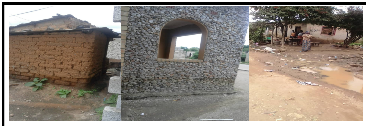
Figure 27: Some of the different materials (mud, stones, bricks) used in the constructions of houses in Kalingalinga slum settlement, 2019.
