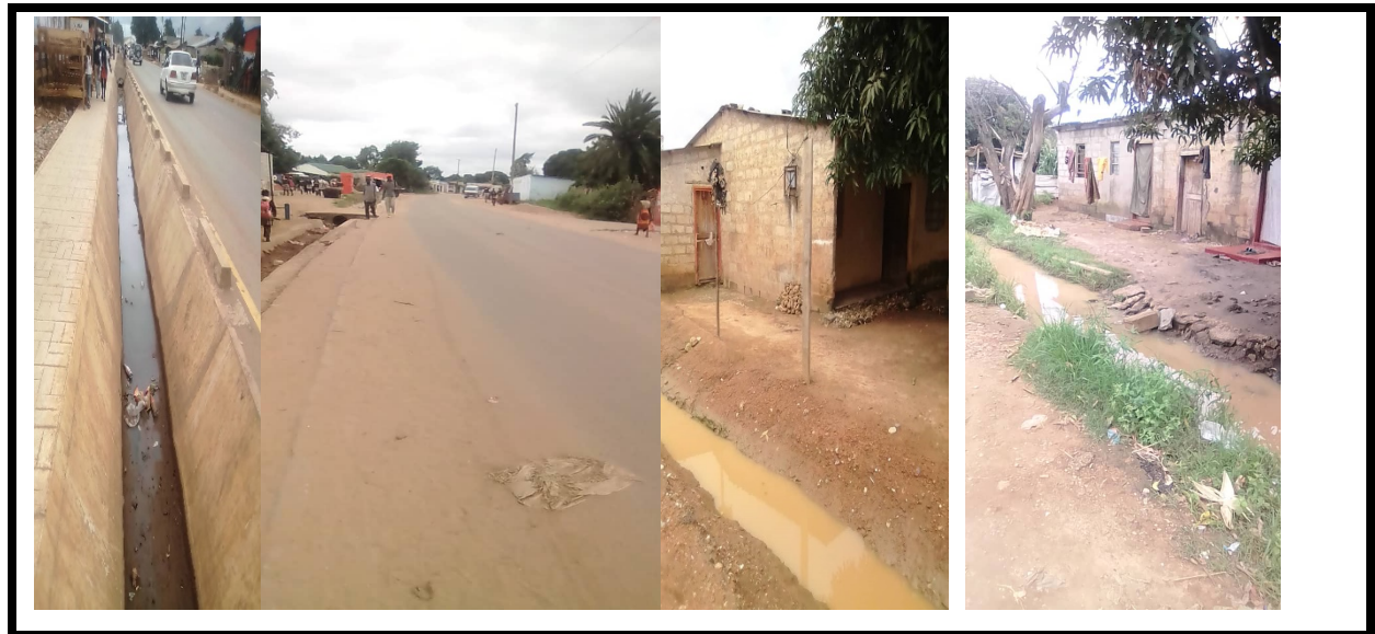
Figure 37: The drainage infrastructure in Kalingalinga, with the two leftmost constructed by government (one cleared of sand and the other blocked). The next two drainages from left are manually constructed and waterlogged.
