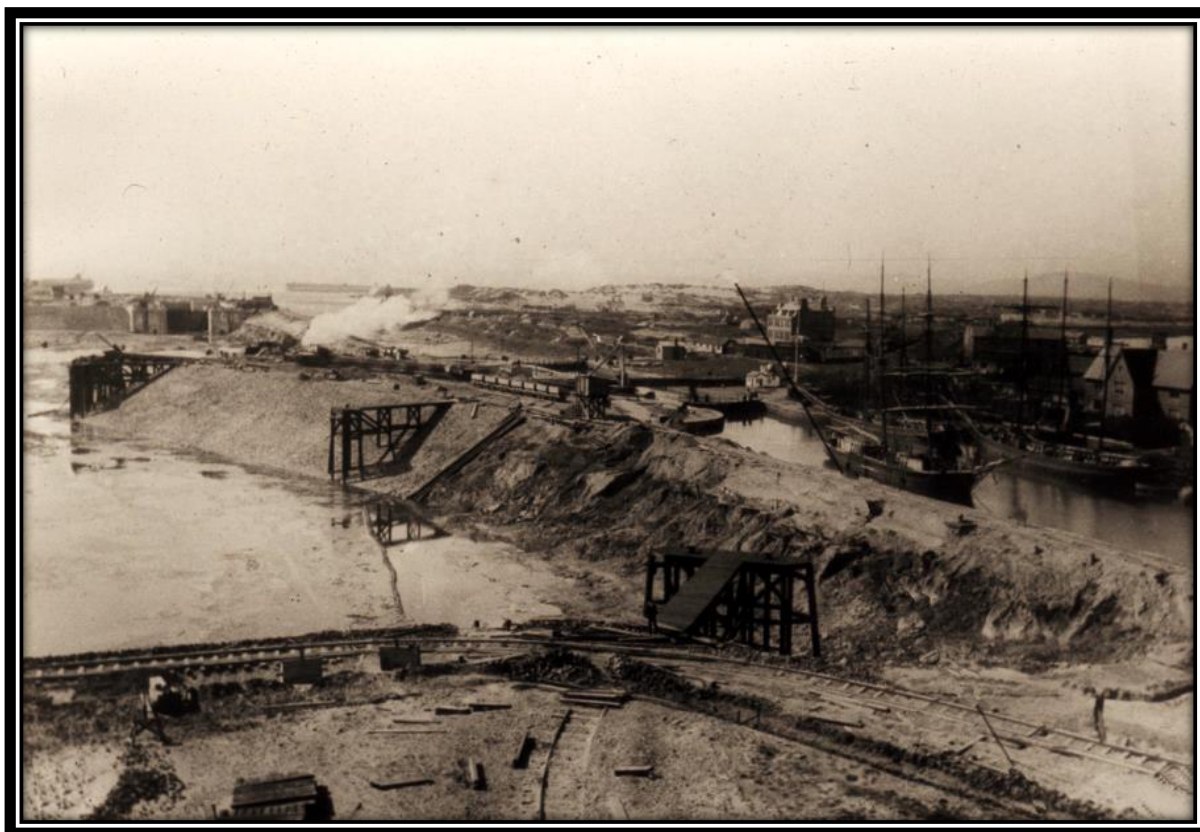
Image 5: Construction of the new docks in 1898
