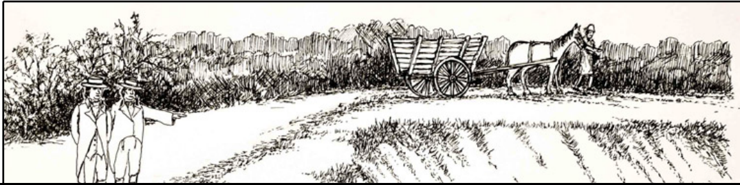
Figure 3 The construction of an eighteenth-century canal: the Fourteen Locks (Newport) 35
