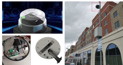
Figure 11. LiDAR hardware installation.
