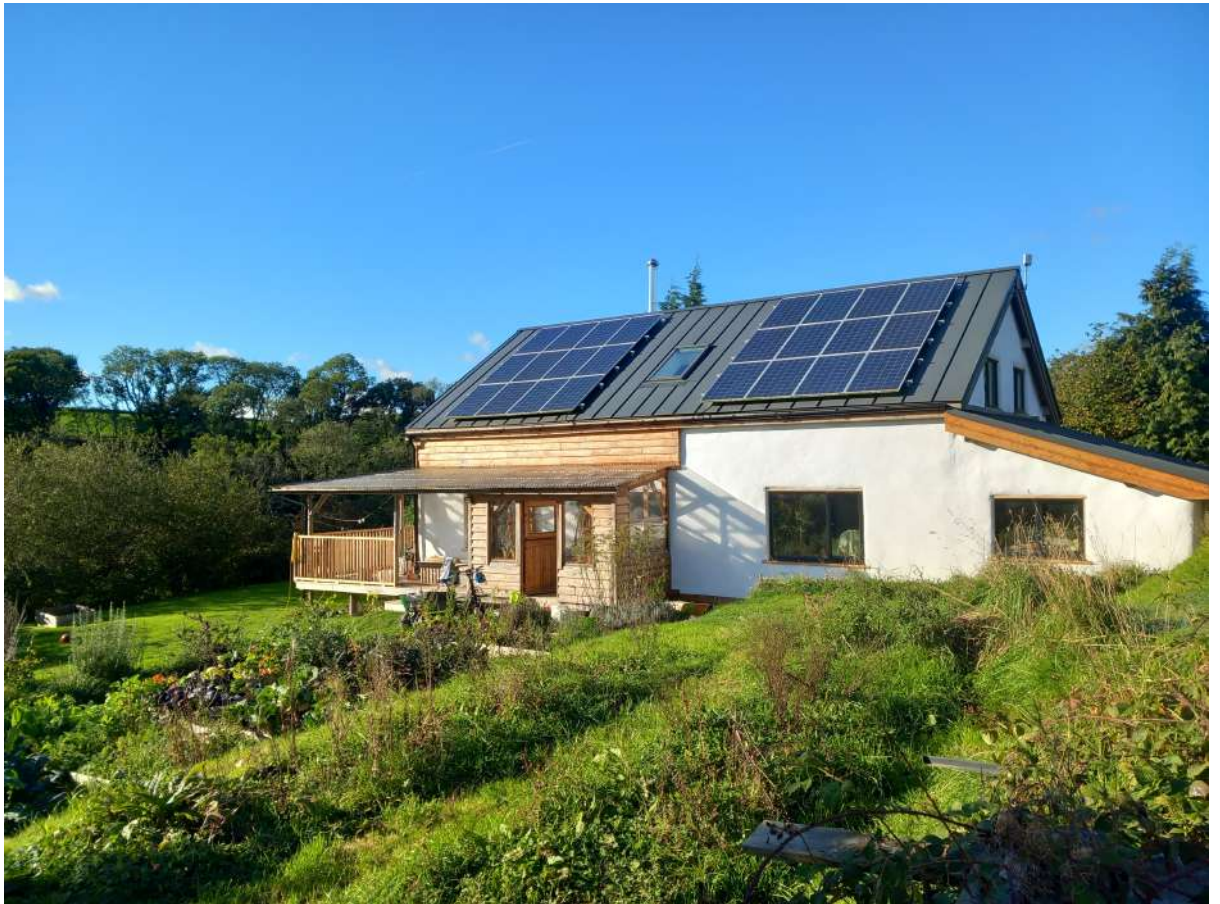
Figure 1. ‘Conventional looking’: Dan Y Berllan OPD has a lime plastered exterior with local larch cladding, large solar arrays cover most of the roof to maximise energy production.
