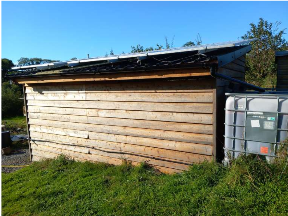
Figure 4. An outbuilding with more Solar Panels, rainwater harvesting, and water storage tank. Water pressure is created using the natural gradient of the land.
