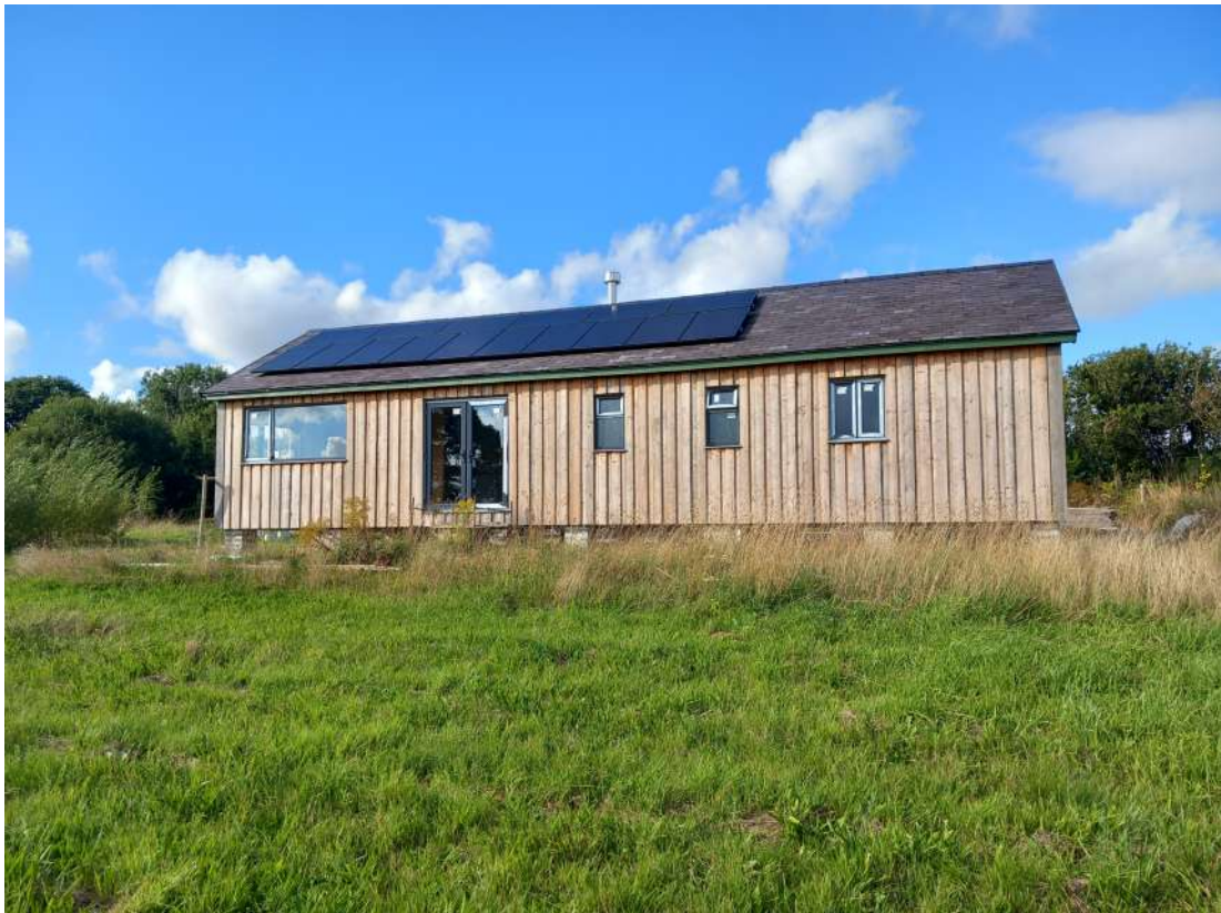
Figure 8. The participants say the house is partly based on a Welsh longhouse and is simple and modest in its design. It is still under construction but is beginning to take shape. It is lifted off the ground to limit the amount of concrete needed as footings,
