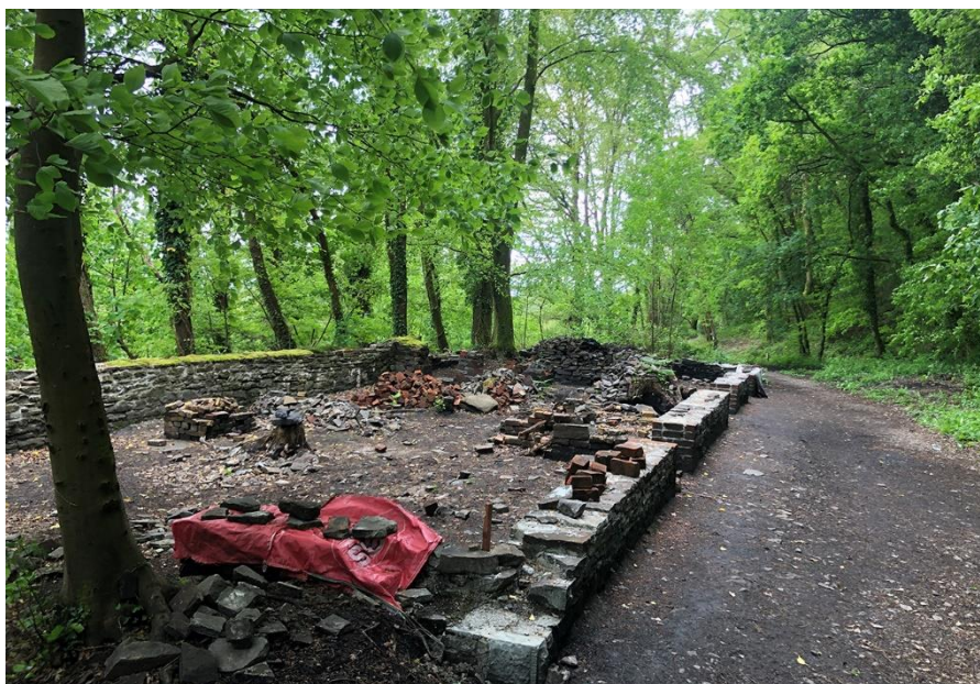
The Victorian colliery smithy site in May 2024 showing new quoin stone in foreground corner and moss-capping left centre © Lisa Kirman
